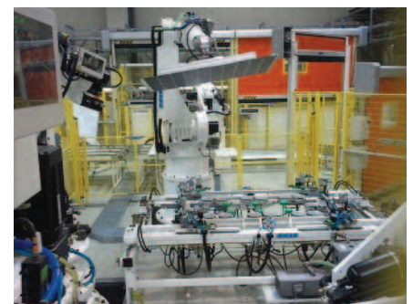
Laminated panel being placed by a robot onto a stand to be framed in aluminum
