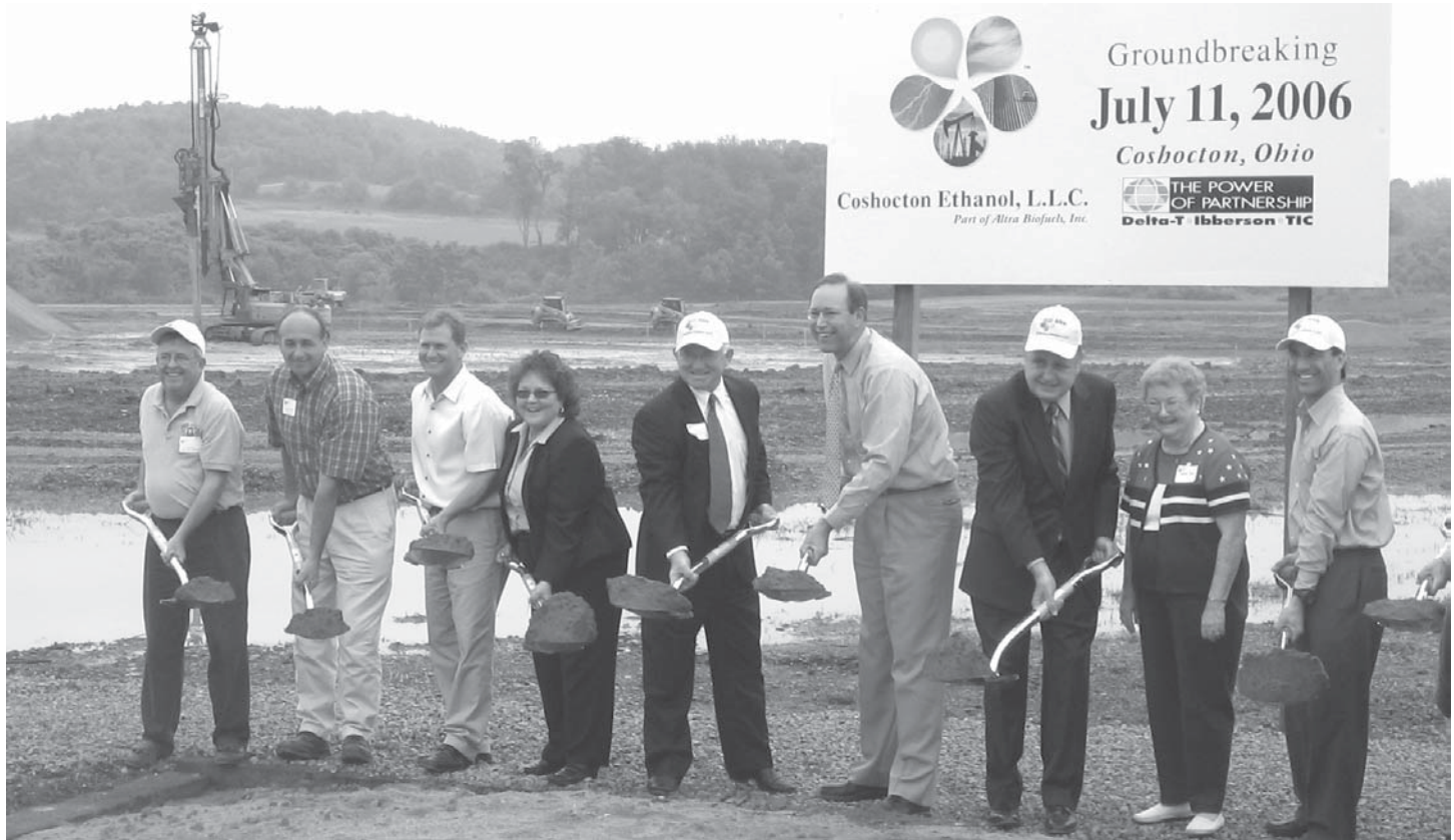
Governor Bob Taft is joined by state dignitaries as he leads the groundbreaking for the new ethanol plant in Coshocton. Clifford R. Cloud, chairman of the OAQDA, is pictured to the right of the Governor.
