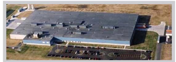
Willard and Kelsey Solar Group Facility
