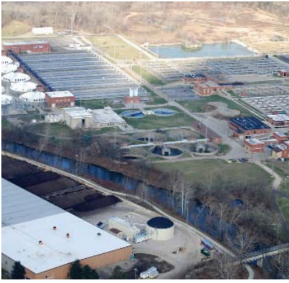
Anaerobic digester system in Akron
